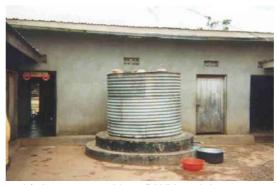
Figure 3: a) An owner built brick tank in Sri Lanka. b) A corrugated iron RWH tank in Uganda.
