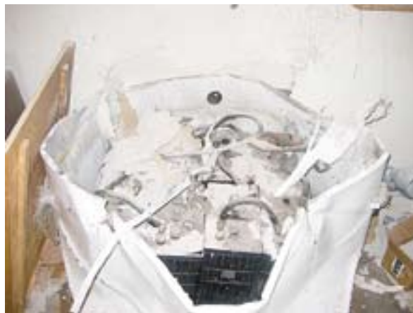
An extreme result of battery neglect.
