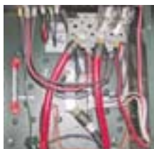
Use bus bars to parallel multiple series strings.
